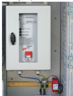
Figure 7 Voltage-controlled short-circuiter VCSD 40 IP65.
